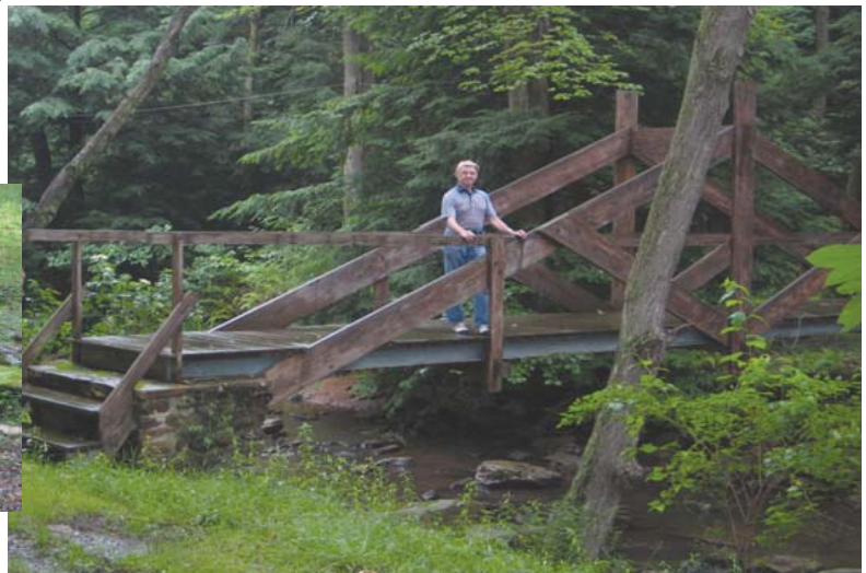
Man-made bridge, redone in 1970
